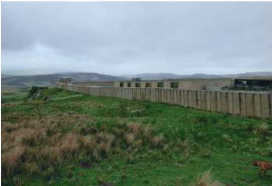
The Forward Operating Base, with views across the Northumbrian hills
